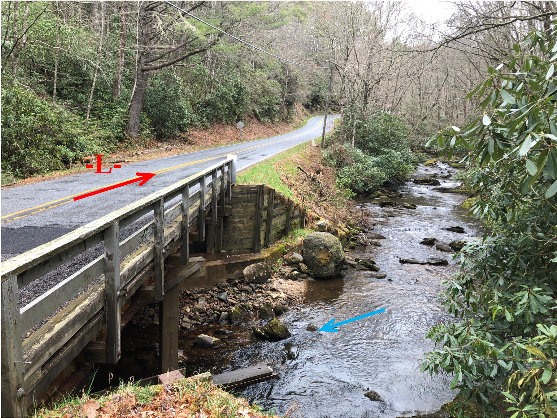
Looking East towards End Bent 2
